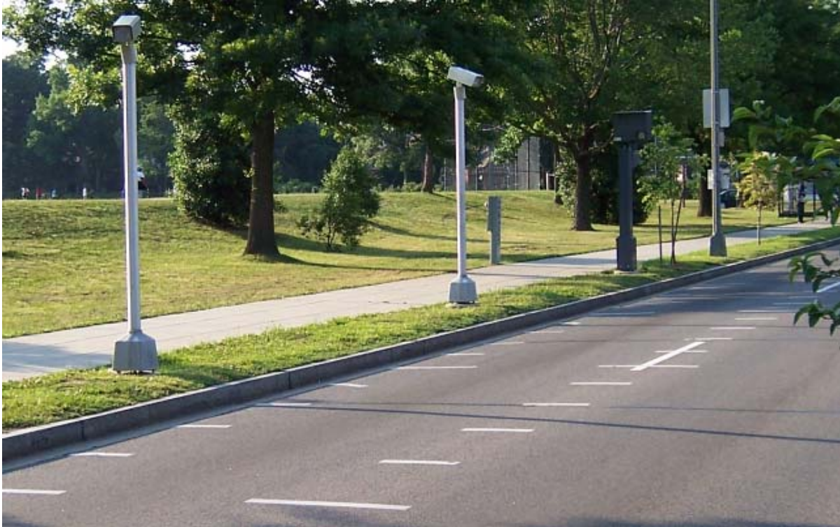
Figure 2. Pole-mounted ASE system in Washington, DC
