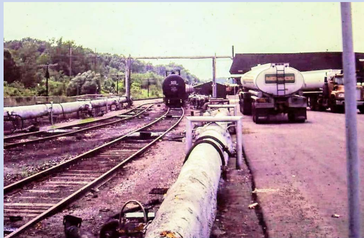
A view of the Monoco asphalt operations in 1984.
