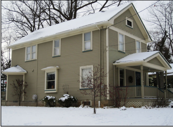
This Foursquare home has been enlarged with a compatible rear wing. A trim board identifies the limit of the original house.
