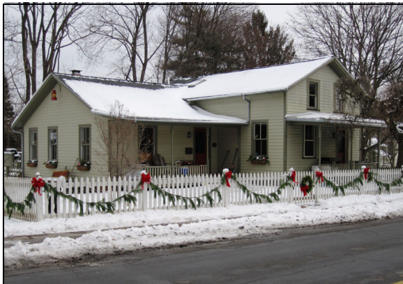
The wing added to this early nineteenth-century home matches the window design and spacing, porch details, and roof form of the original house.
