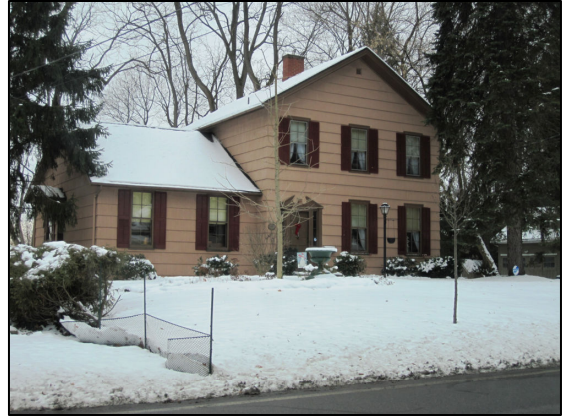
This mid nineteenth-century home has a new side wing. The wing matches the window size and other details of the original house. The main block with side wing massing is typical of mid nineteenth-century vernacular homes.
