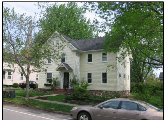
This ca. 1910 Four-square house was enlarged with a side wing. The wing respects the simple design, roof slope, window style, void-to-solid-ratation and proportions of the original house.
