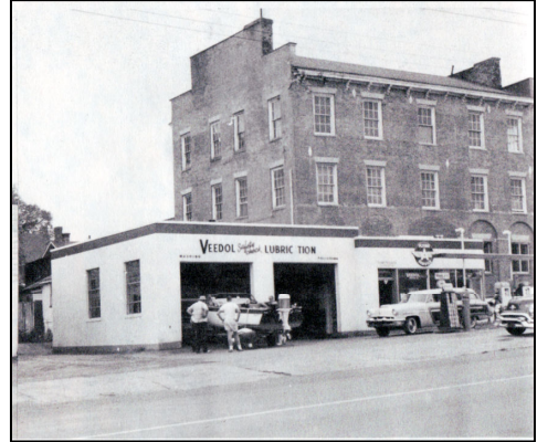
In 1957, before the Village's preservation ordinance was adopted, a gas station was constructed disfiguring the main facade of the Phoenix Building.
