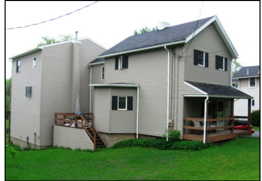
This house in a neighboring village has lost its historic character due to poorly designed additions and alterations.
