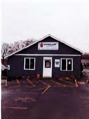
Front view of Building G
