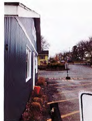
View from front east corner toward Route 31, Schoen Place
